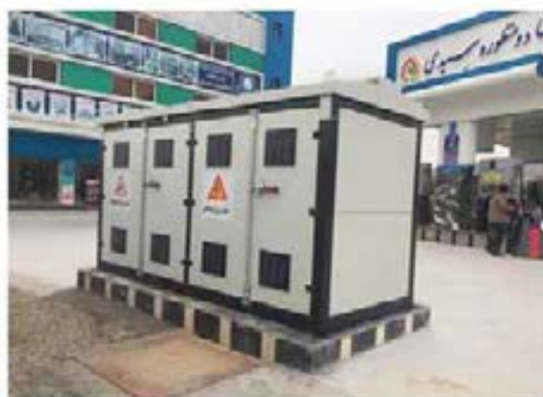
Kiosk Substation Capacity : 100 up 2500 KVA Voltage : up to 36 KV
